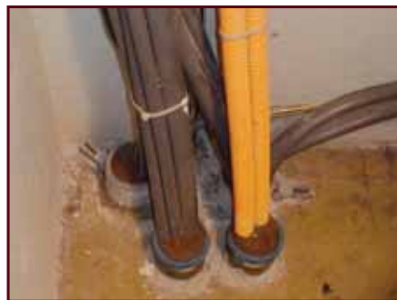
Kwikpath Riser lets you run communication cables effortlessly from floor to floor through vertical shafts.
