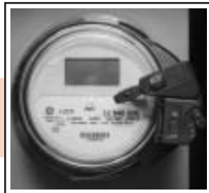
Electronic Meter Front Optical Port AT LEAST 1½ inches from outer rim of dome. If in doubt, physically measure the distance.
